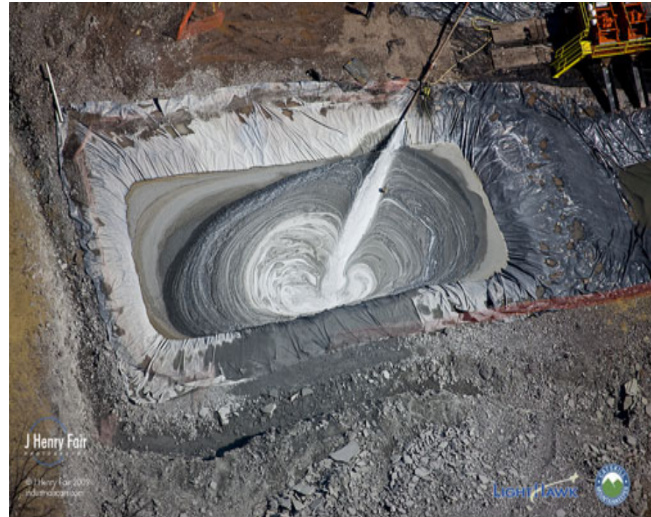
(Drilling fluid splashing past the liner, Dimock, PA, Spring 2009)
