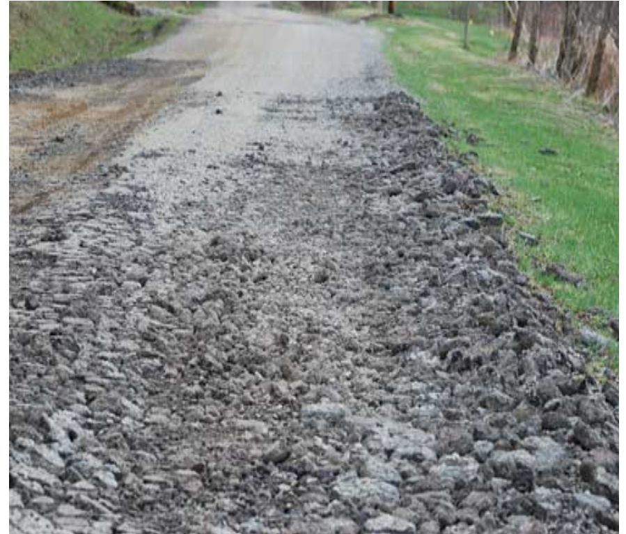
Road damage on secondary blacktop.
