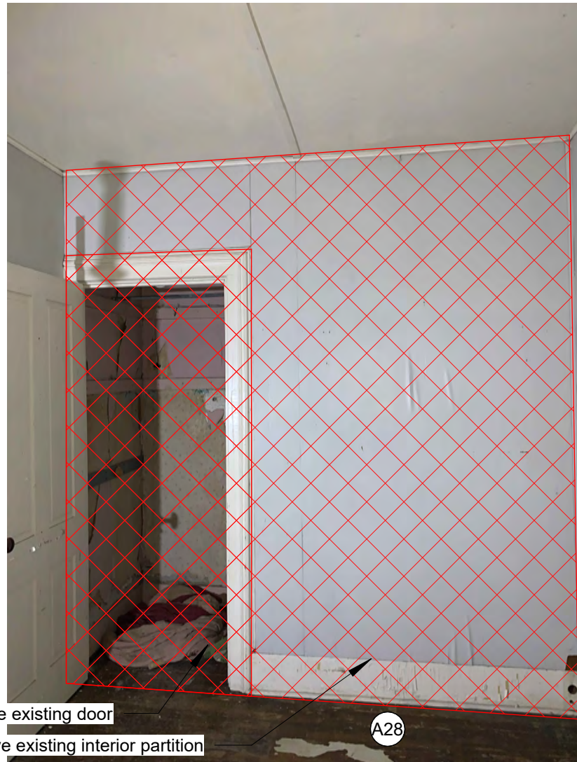
6 Second Floor Existing Photo 06 NOT TO SCALE
