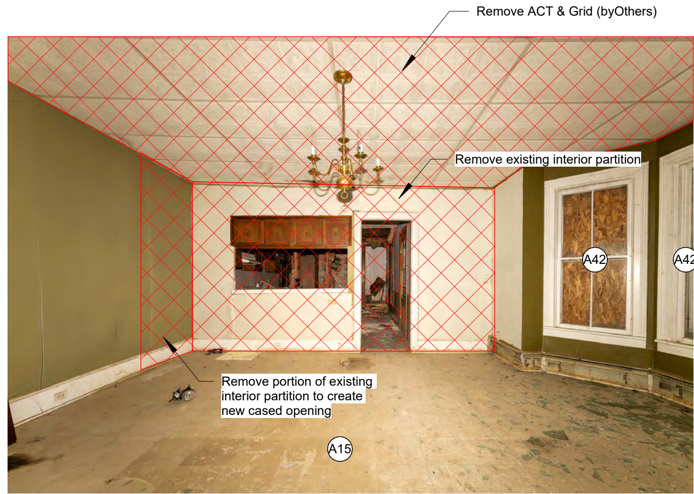
8 First Floor Existing Photo 04 NOT TO SCALE
