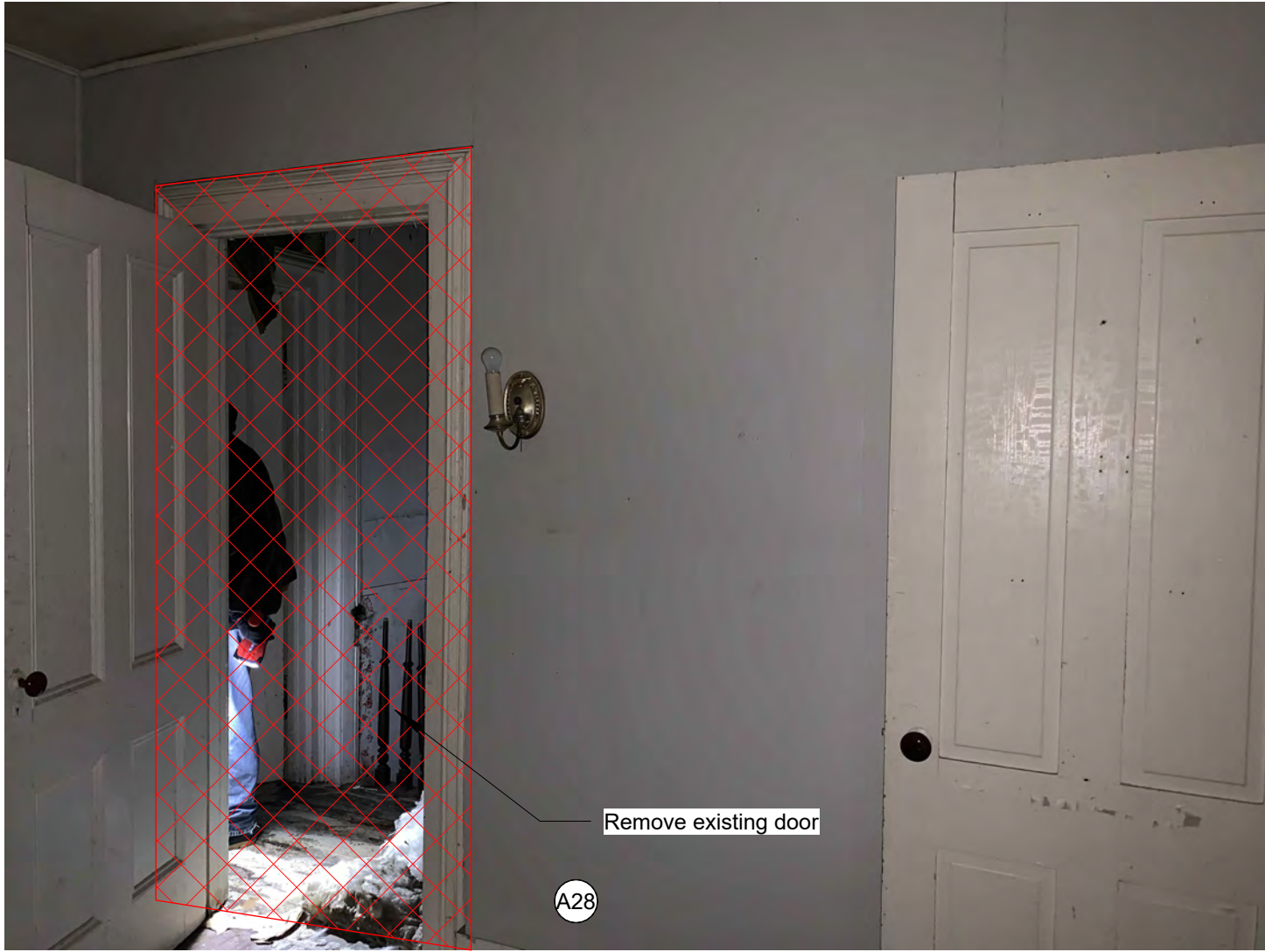
7 Second Floor Existing Photo 07 NOT TO SCALE
