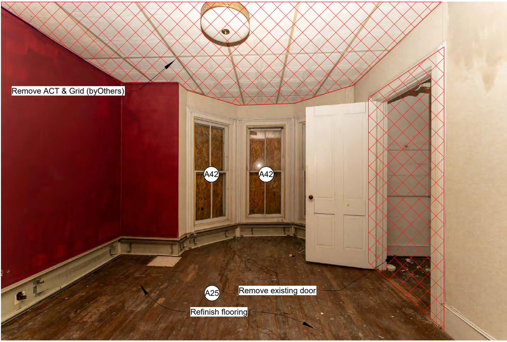
8 Second Floor Existing Photo 08 NOT TO SCALE
