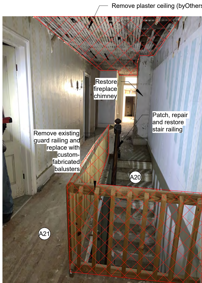
1 Second Floor Existing Photo 01 NOT TO SCALE
