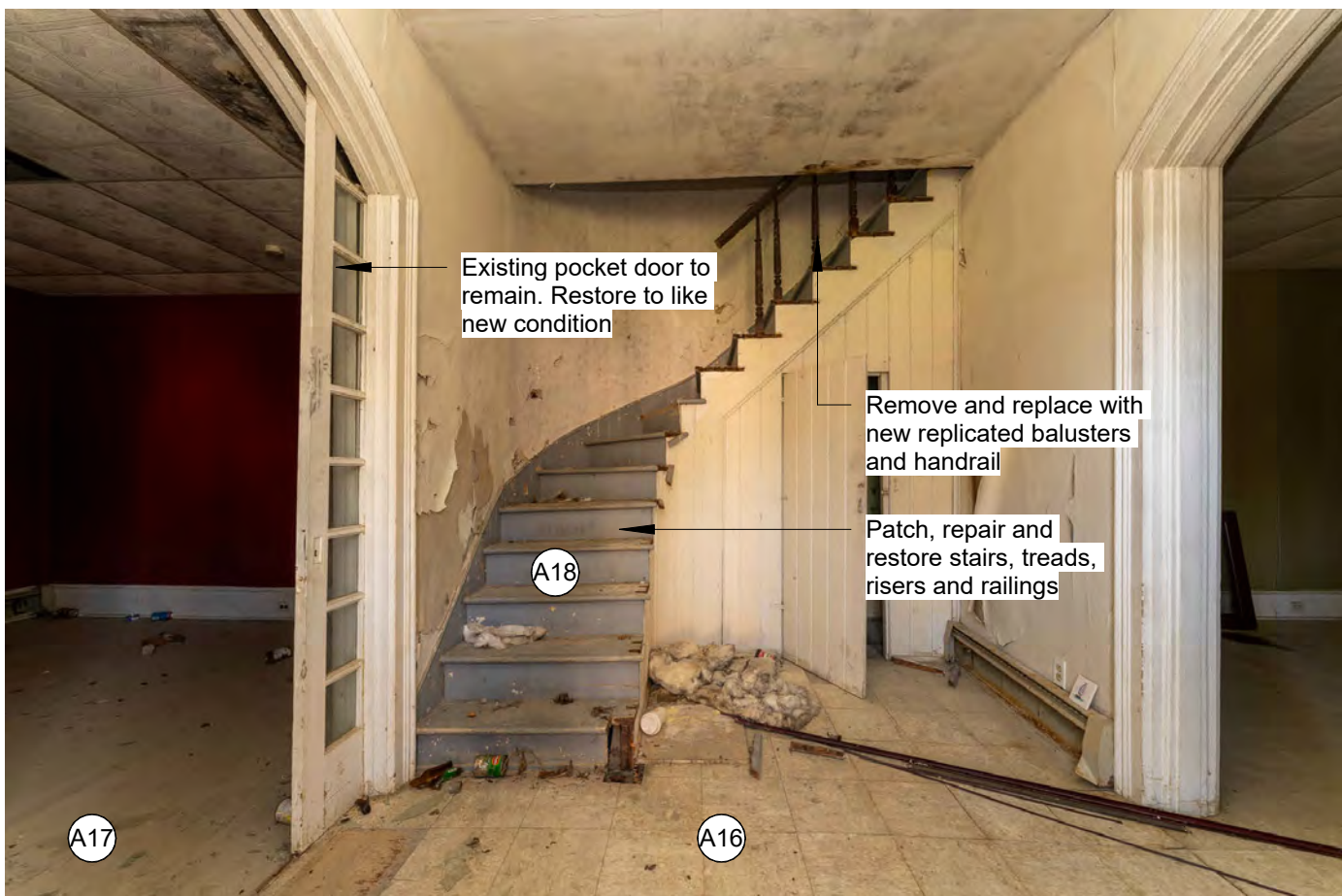
6 First Floor Existing Photo 02 NOT TO SCALE
