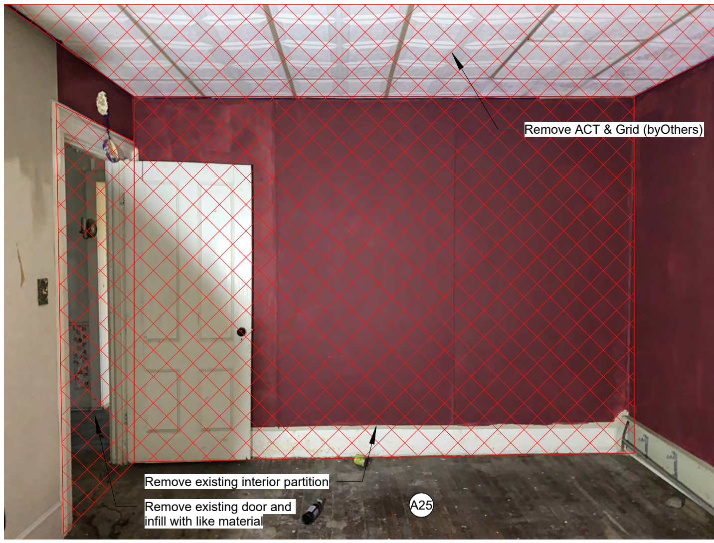
9 Second Floor Existing Photo 09 NOT TO SCALE
