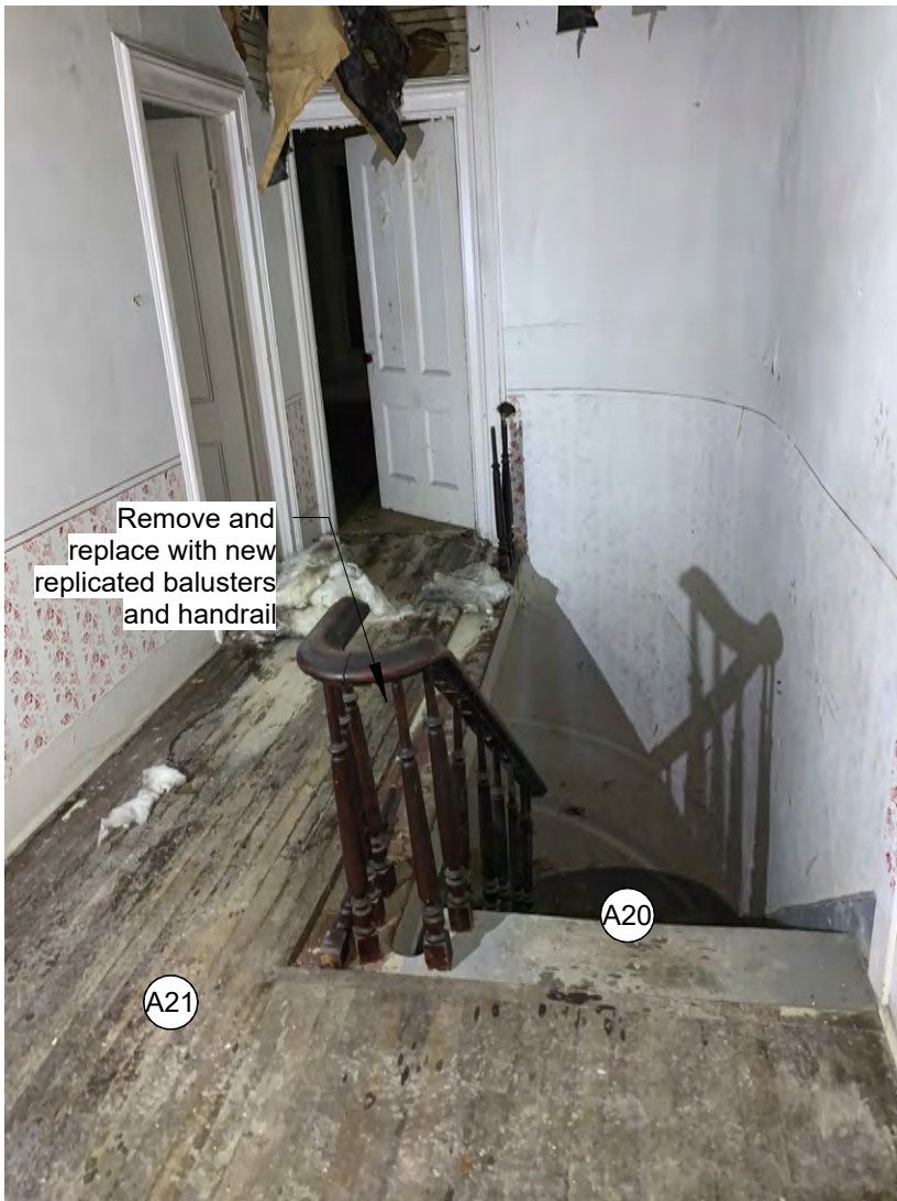
2 Second Floor Existing Photo 02 NOT TO SCALE
