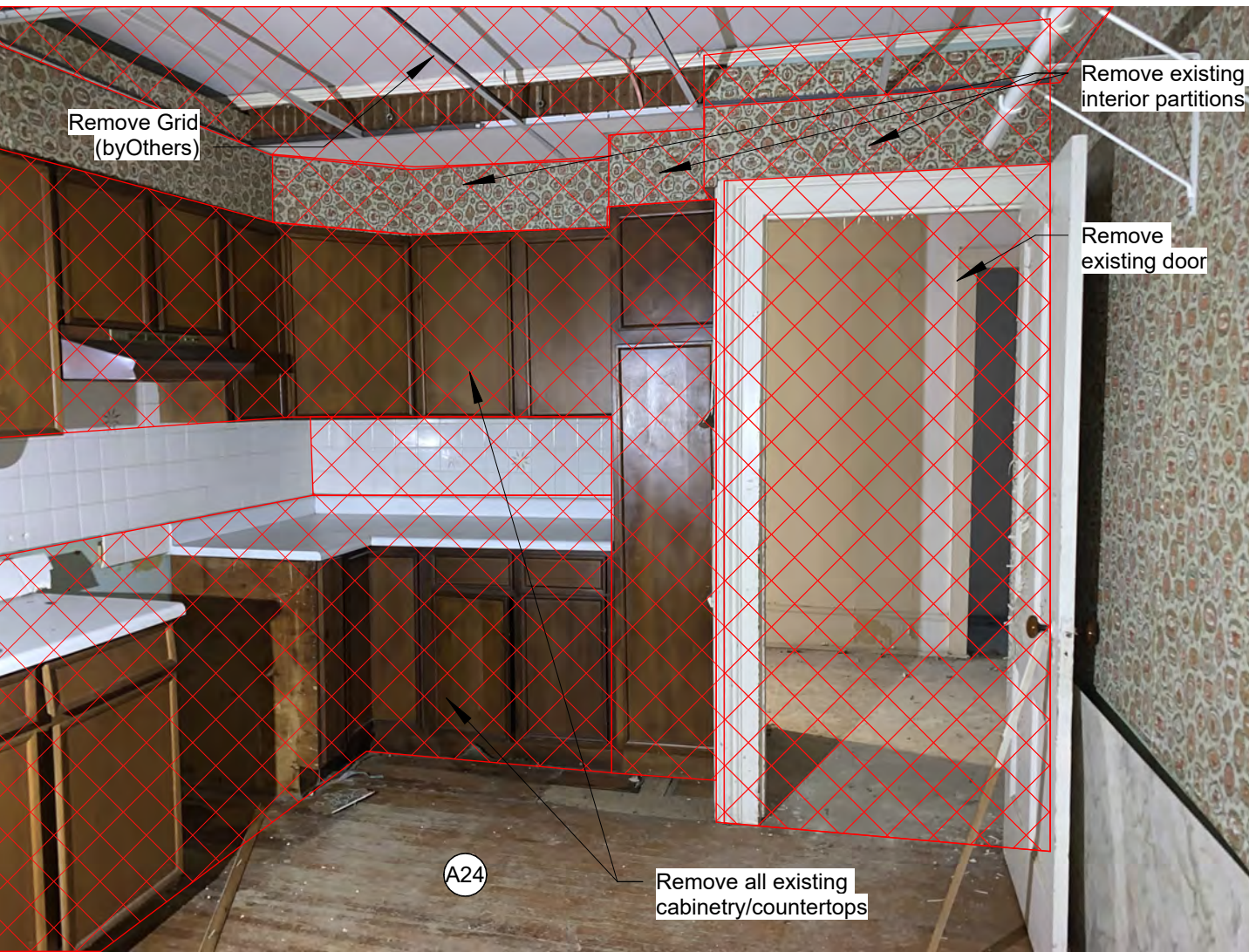
10 Second Floor Existing Photo 10 NOT TO SCALE
