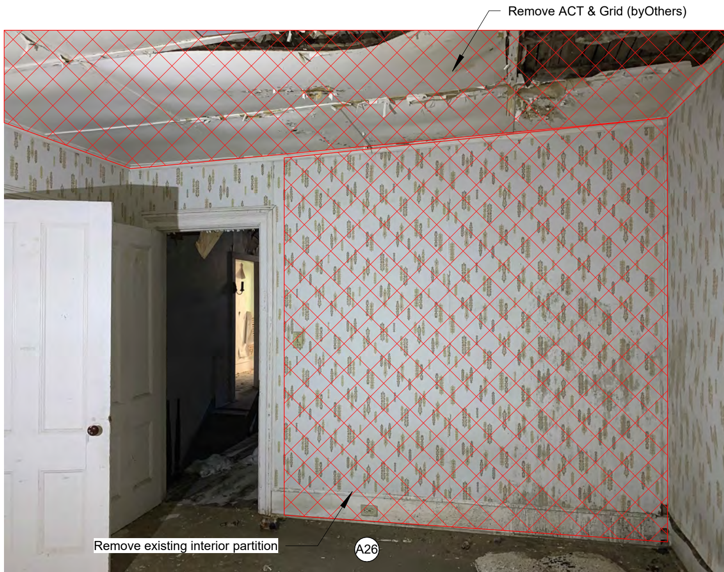
3 Second Floor Existing Photo 03 NOT TO SCALE
