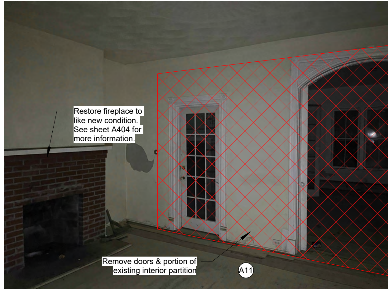
12 First Floor Existing Photo 08 NOT TO SCALE
