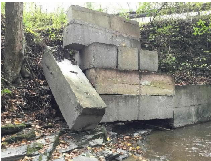
Allen Glen Road over Huntington Creek. Severely unstable wingwall upstream of structure inlet.
