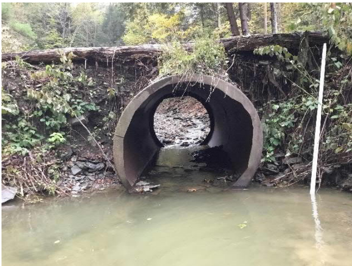
Private Driveway off Dean Street over Huntington Creek (upstream). Crossing structure outlet. Note erosion of road embankment on either side of structure.
