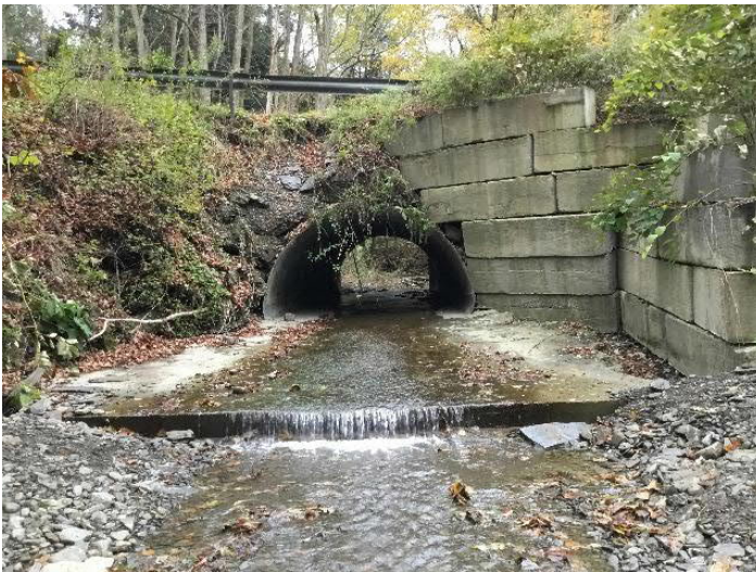
Allen Glen Road over Huntington Creek. Structure outlet. Note unstable wingwall and concrete-lined streambed, eroding road embankment, and outlet drop.
