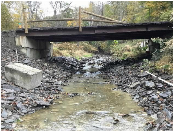
Private Driveway off Dean Street over Huntington Creek (downstream). Structure inlet. Note sagging abutment and displaced concrete waste block on left bank.
