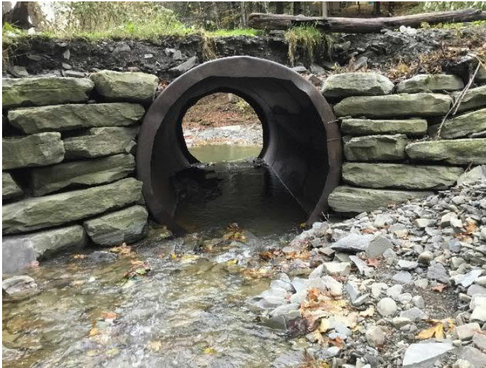
Private Driveway off Dean Street over Huntington Creek (upstream). Close-up photograph of structure inlet. Note inadequate fill/cover material above culvert, erosion of road along top of structure, and sediment deposition on river right.
