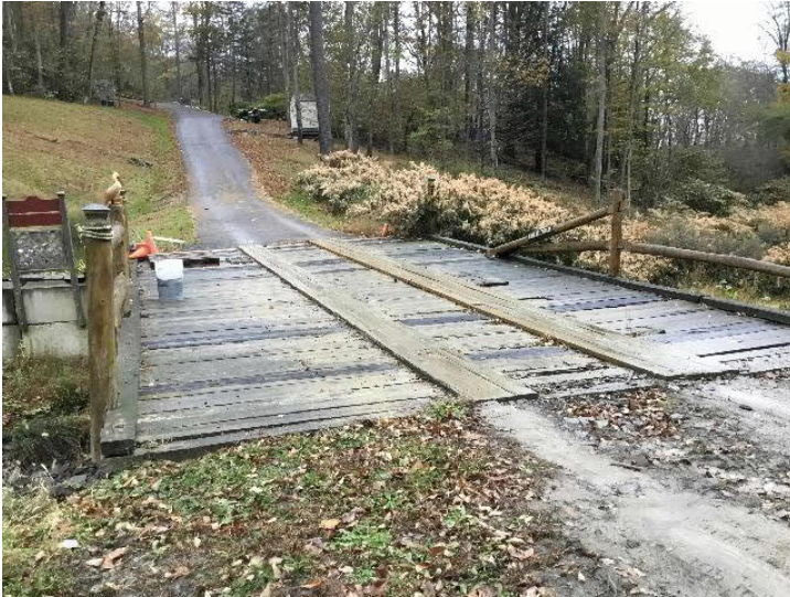
Private Driveway off Dean Street over Huntington Creek (downstream). Photograph of bridge deck. Note planks placed lengthwise on bridge deck to support vehicle traffic.
