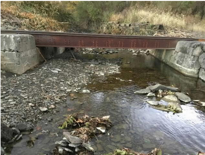
Outlet of Owego & Hartford Railroad bridge over Huntington Creek. Note low bridge clearance, constriction of stream by bridge abutments, and timber retaining wall lining upstream channel.
