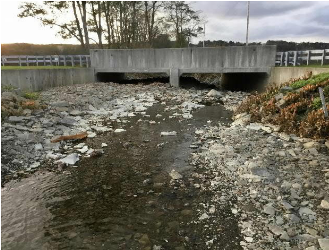
Inlet of Sheldon Guile Boulevard crossing over Huntington Creek. Note sediment nearly filling culvert structures.
