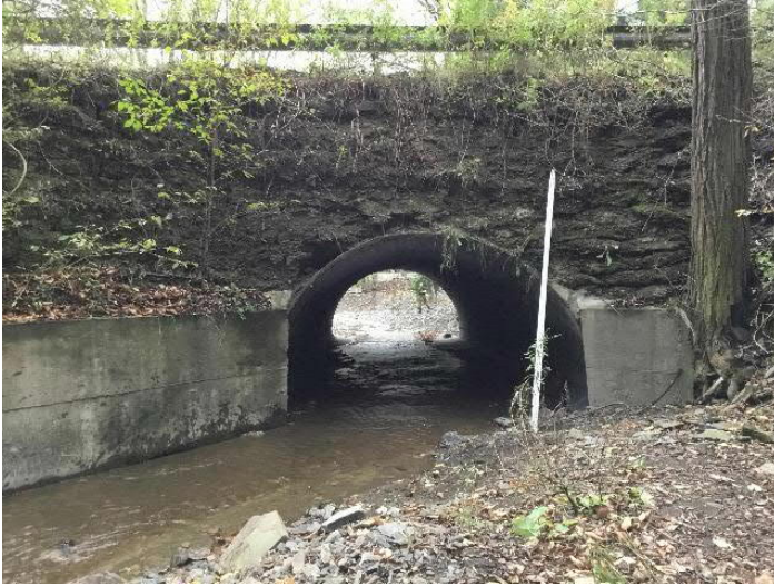
Allen Glen Road over Huntington Creek. Structure inlet. Note missing headwall exposing embankment formed of stacked bags of grout.
